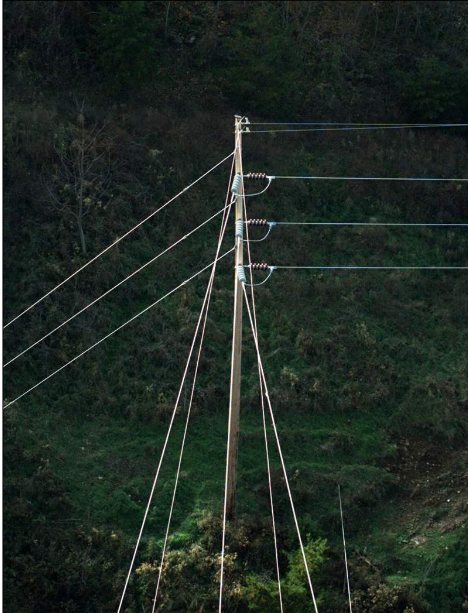
COMPARABLE EXISTING STRUCTURE PHOTOGRAPH
