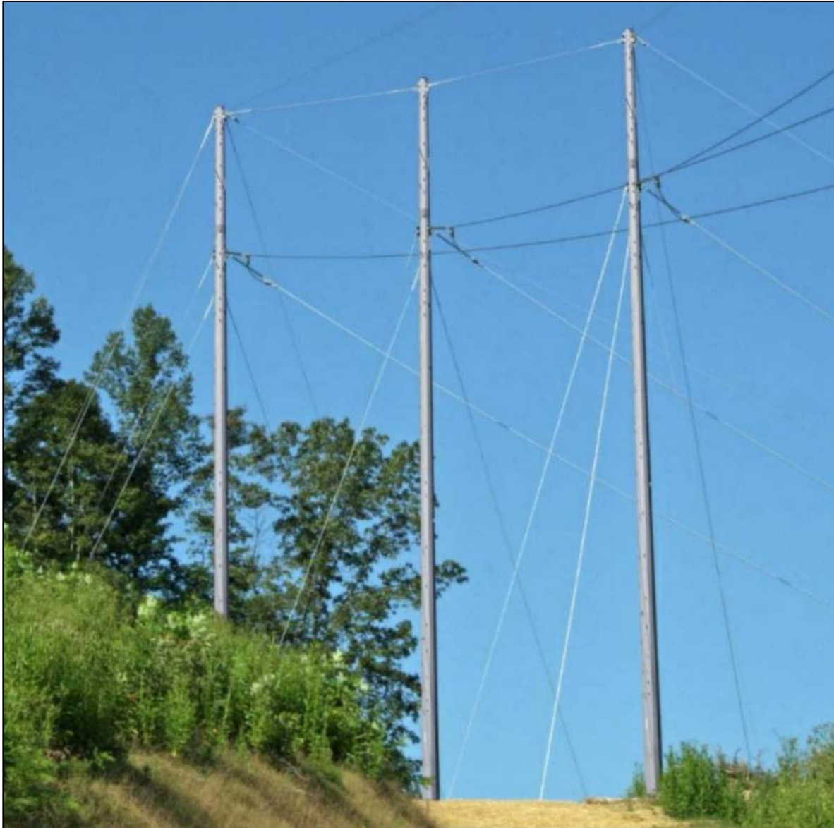
COMPARABLE EXISTING STRUCTURE PHOTOGRAPH
