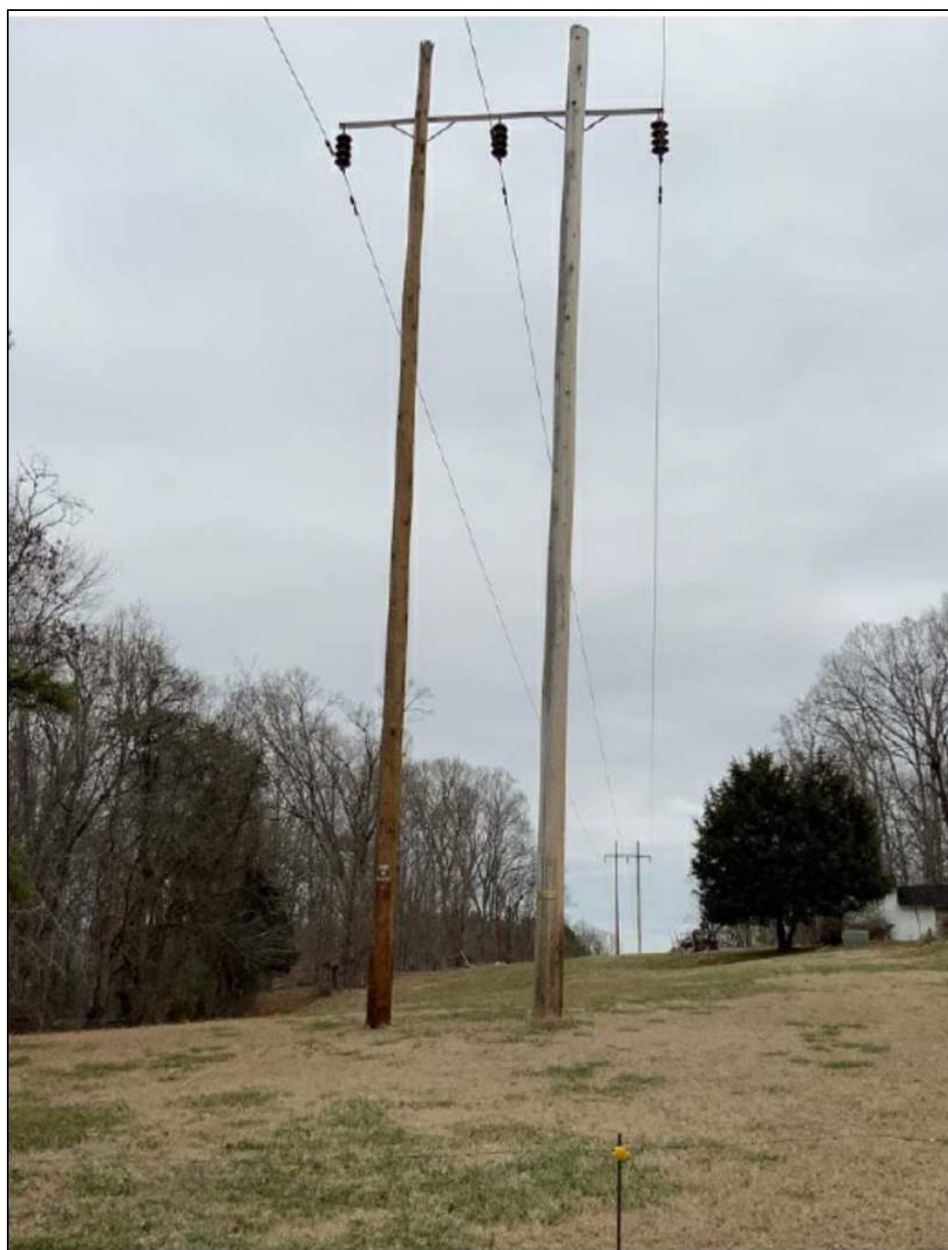
COMPARABLE EXISTING STRUCTURE PHOTOGRAPH
